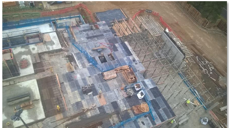
View from Tower Crane - First Floor Slab Formwork in Progress
