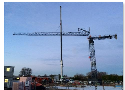
ABOVE: the back jib being lifted onto the mast, onto this the counterweights are installed
