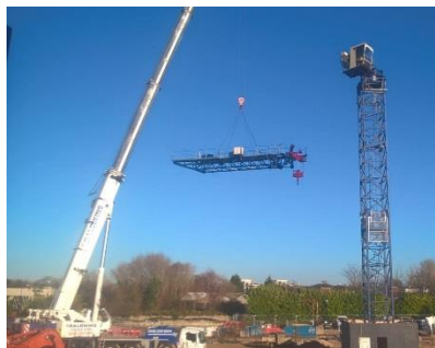
ABOVE: the back jib being lifted onto the mast, onto this the counterweights are installed
