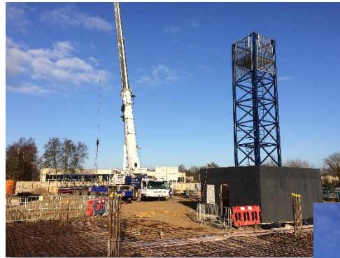
ABOVE: the first section of the mast erected
