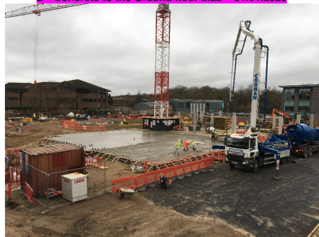
2 nd Concrete to the Ground floor slab – 31.01.2020
