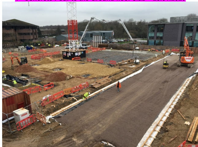
2 nd Concrete to the Ground floor slab – 31.01.2020
