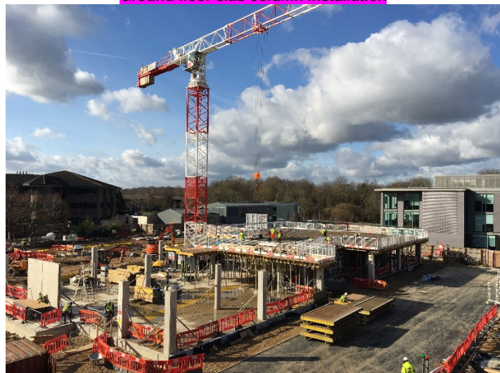
Ground floor slab column installation
