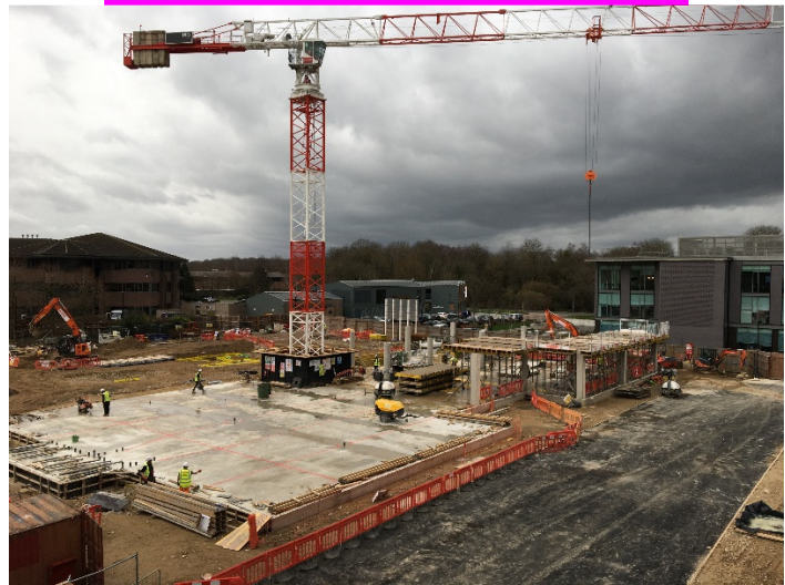
Level 1 Slab Construction Commenced – 03.02.2020
