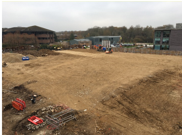
Piling Platform constructed, reading for piling to commence.
