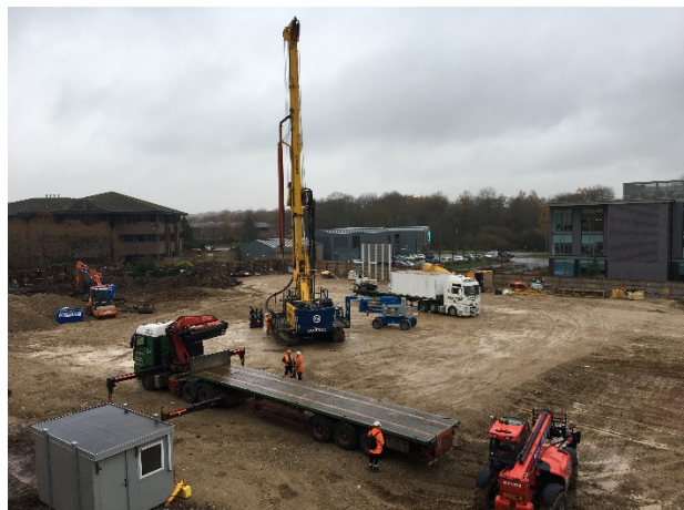
Piling Rig mobilization
