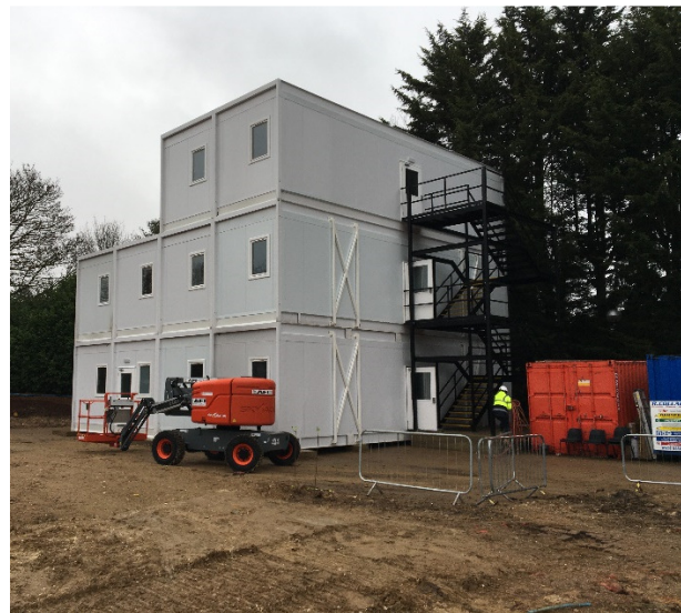
Our New Project Office
