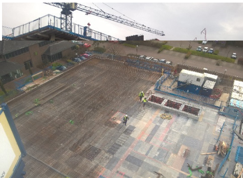
Structure Progress – Entrance Reception Area Preparation for Roof Pour
